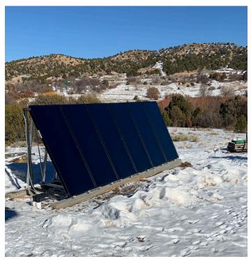
Six beautiful, powerful solar panels filled with glycol to transfer heat from the sun to the water feeding the boiler feeding the underfloor heating in the entire building and the hot water in showers and sinks in the new section.
